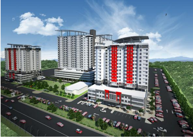
- Car Park System and Access Control System at Calista Block M at Puchong Mas
