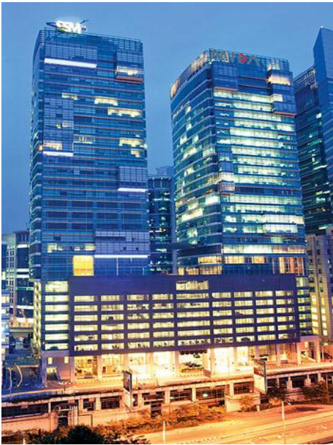
162 Paxton Net2 plus Controllers for Access Control at MIDA building at KL Central
