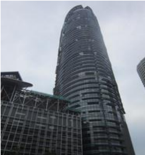
-77 Access Door System at Menara Felda in KL(on Going Project)
